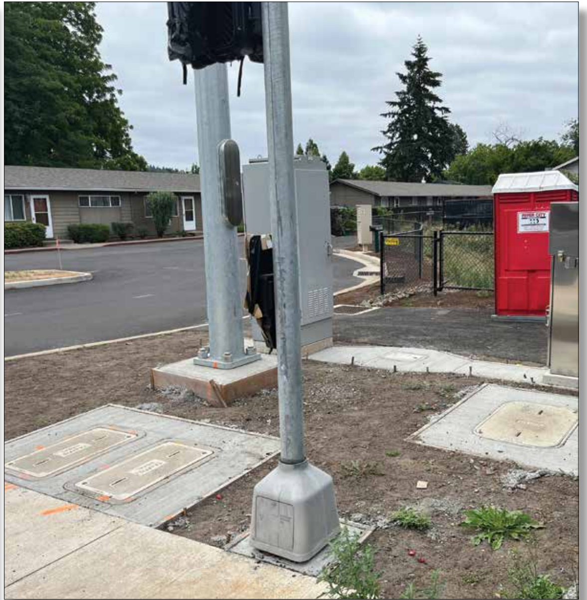
The street areas near Johnson Creek Fred Meyers recieved a major overhaul with this project. Curbing was sha ved and altered to make it much more accessible and definitive for motorists to see people at the crossings. The electrical work was upgraded and replaced completely with much sturdier wiring and signal boxes.
