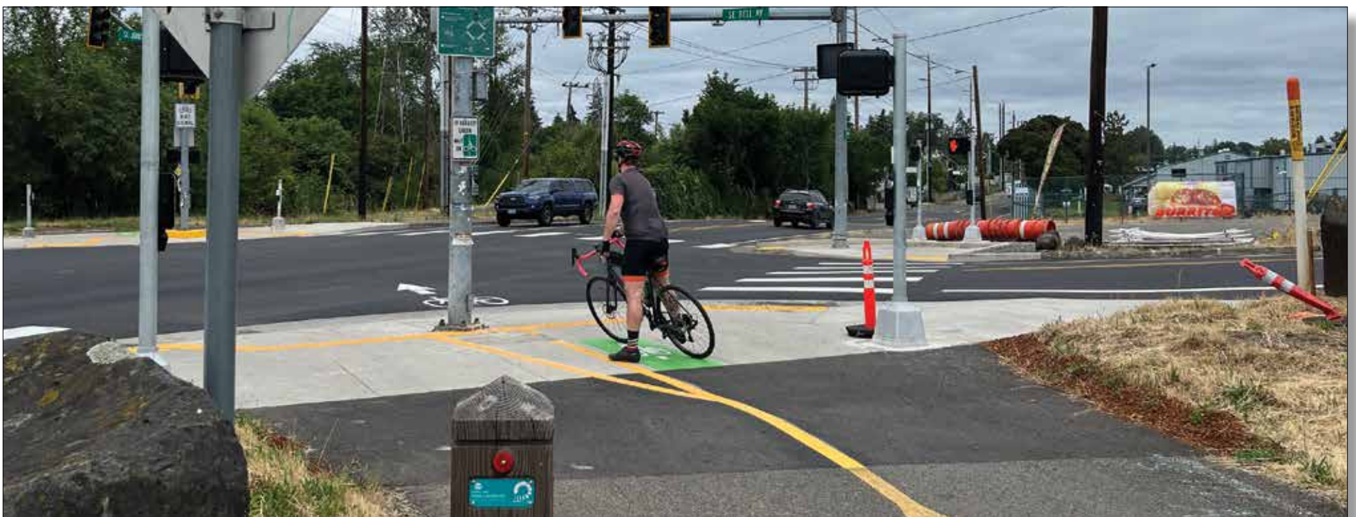
This intersection on Johnson Creek Blvd. and SE Bell Avenue is part of the Springwater Corridor Trail, making an unusual diagonal crossing through the roadways with bike sensors on both sides. Updates include the ramps, sensors and new crossing button poles. PHOTOS BY PAUL NEUFELDT
