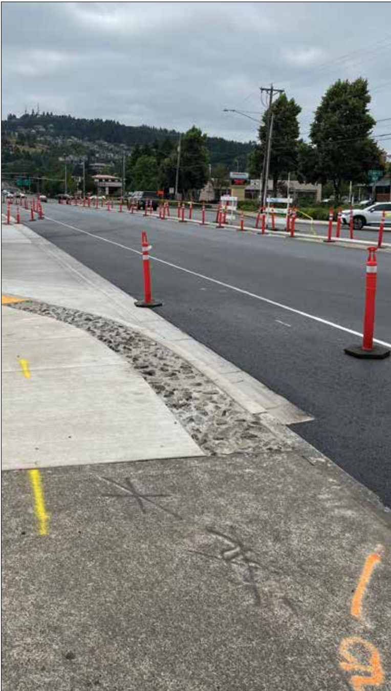
The street areas near Johnson Creek Fred Meyers recieved a major overhaul with this project. Curbing was sha ved and altered to make it much more accessible and definitive for motorists to see people at the crossings. The electrical work was upgraded and replaced completely.with much sturdier wiring and signal boxes.
